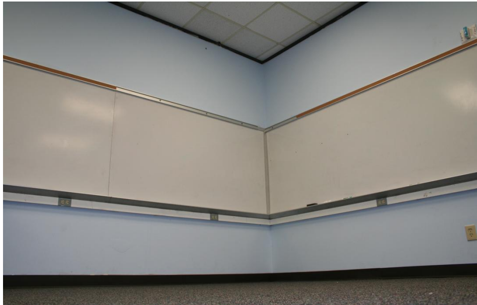
New paint, new white boards, new carpet, and electrical work complete.
